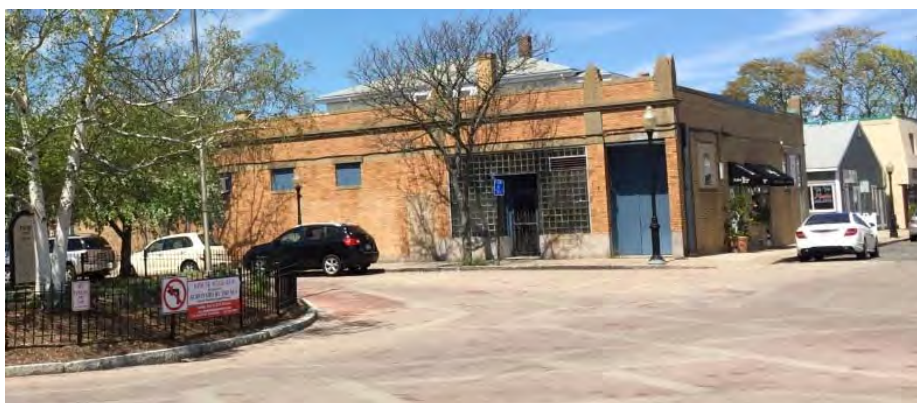
Figure 22. A one-story building fronting on French Square
