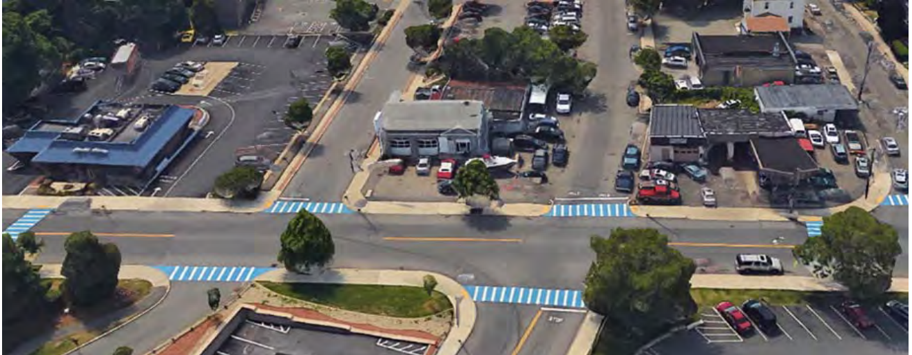
Figure 23. Underutilized parcels line the south side of Pauline Street
