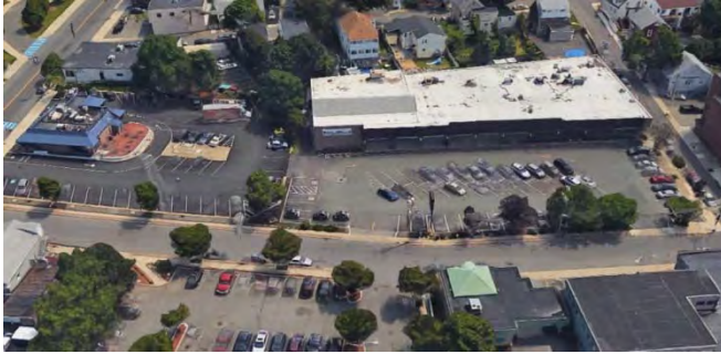
Figure 25. No buildings front on Putnam Street between Pauline & Jefferson Streets
