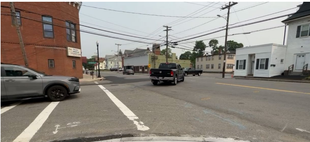
The intersection of Bay St and Britannia St is one of the busier intersections in Whittenton, providing critical east-west access between Washington St and Broadway and the Reed & Barton Complex.
