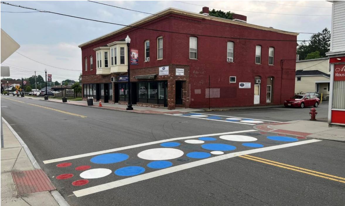
The completed tactical design intervention at Bay St. and State St. (Photo Credit: City of Taunton)
