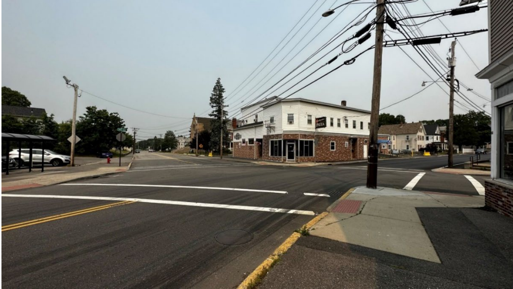
The irregular shape of the intersection at Bay St and Whittenton St creates unsafe conditions for all users, including high speed turns and poor visibility.
