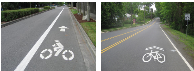
Below: On secondary and feeder streets, on-street bike lanes or shared lane markings help bicyclists to feel more comfortable and to encourage bicycle commuting.
