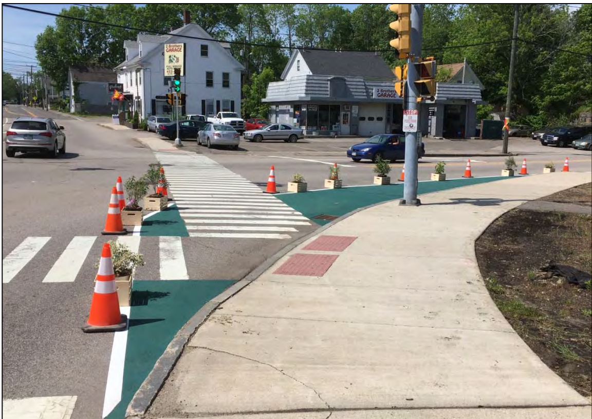
Figure 15. Example of Temporary Curb Extension Used to Test Feasibility.
