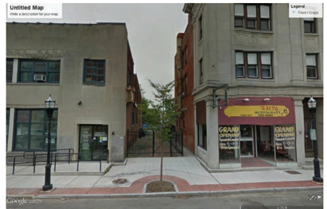
Existing conditions of entrance to the alleyway.
