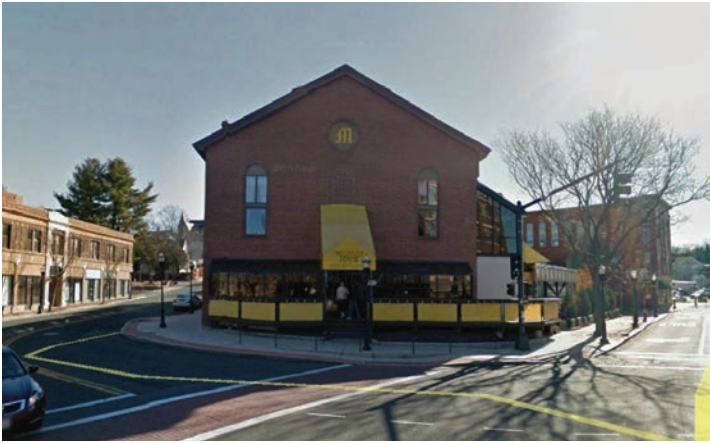
Munich Haus on Center Street
