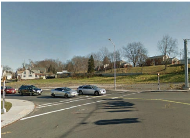
Center and Hampden Street intersection.
