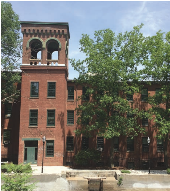
The Ames Manufacturing building is being converted into residential condos.
