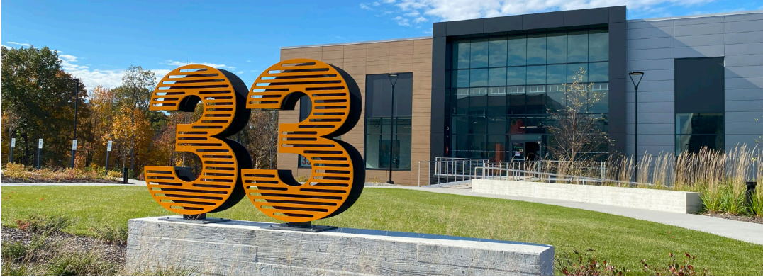
Electric Hydrogen's new facility at 33 Jackson Road
