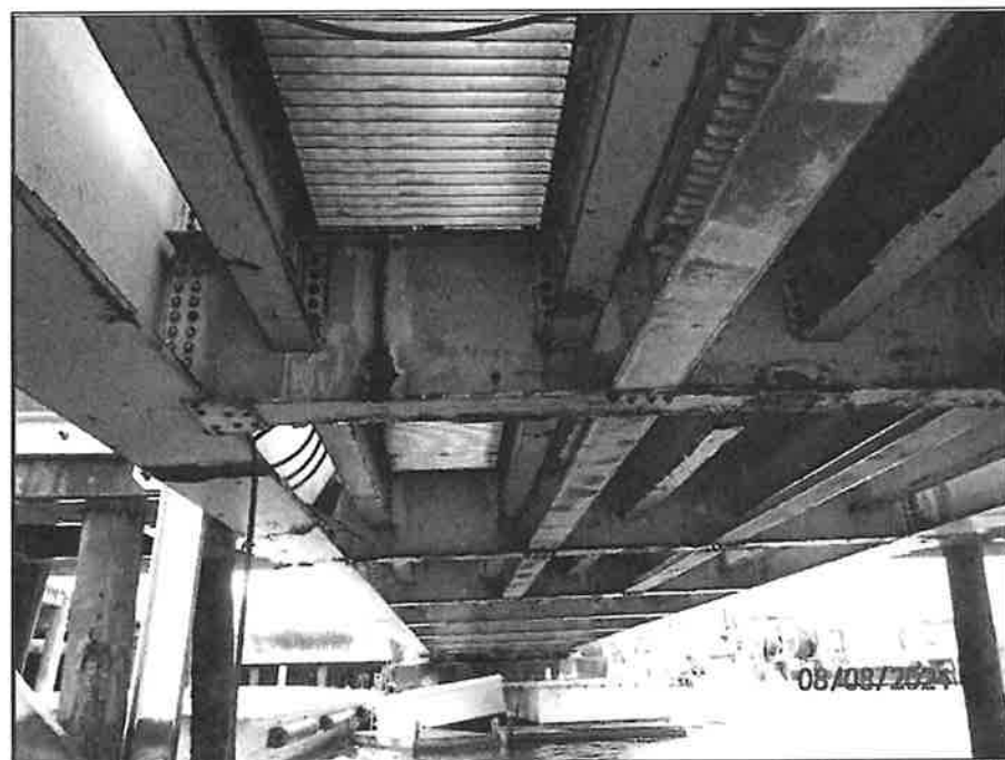
Photo 8 –Underside of Ramp Superstructure (looking west)
