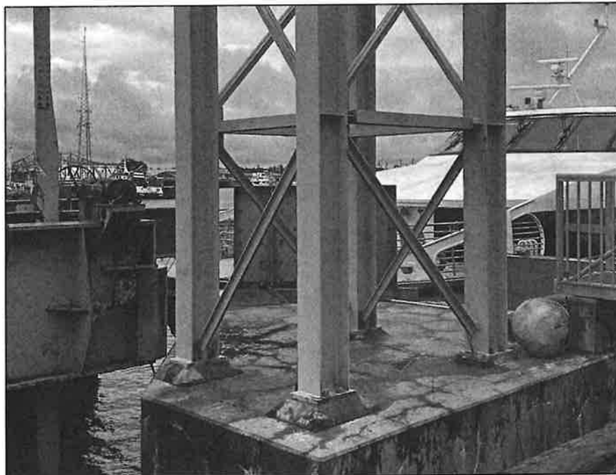
Photo 18 – View of Southeast Hoist Tower Base
