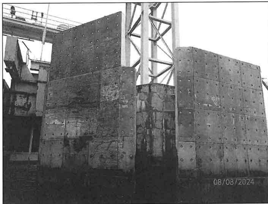
Photo 3 – Typical Dolphin Fender Condition (north dolphin shown)
