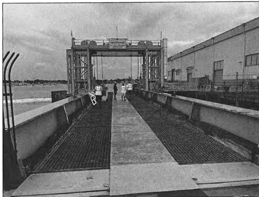
Photo 2 –Topside of Ramp (looking east)
