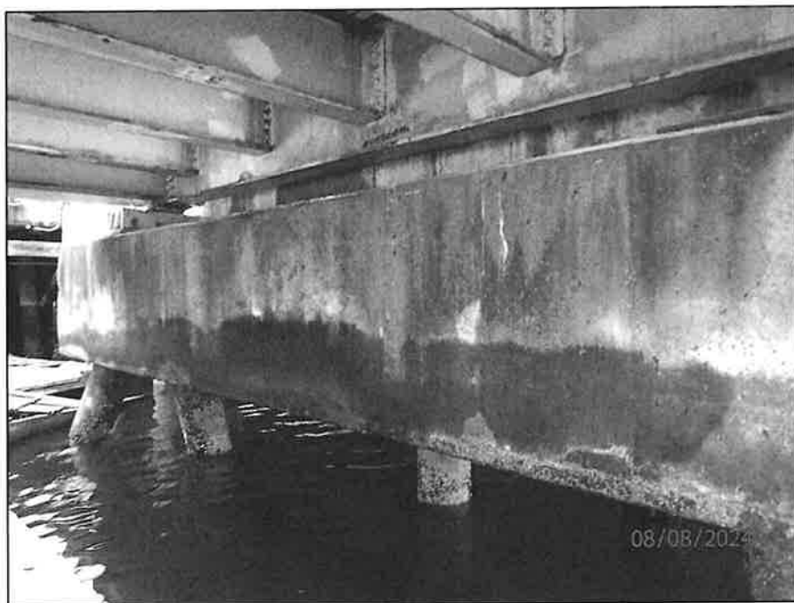
Photo 12 – Abutment Elevation (looking southwest)
