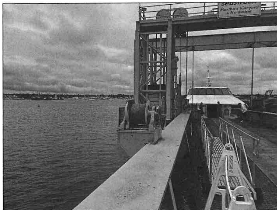
Photo 20 – Cable reel mounted to the north girder
